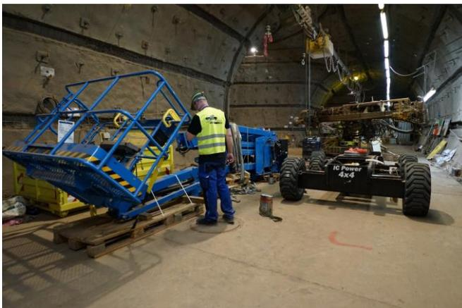
*Only accessible via elevator, the Genie® Z®-45 XC™ boom lift was dismantled and reassembled inside the pit.*
